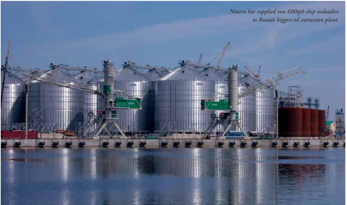
*Neuero has supplied two 600tph ship unloaders to Russia's biggest oil extraction plant.*
