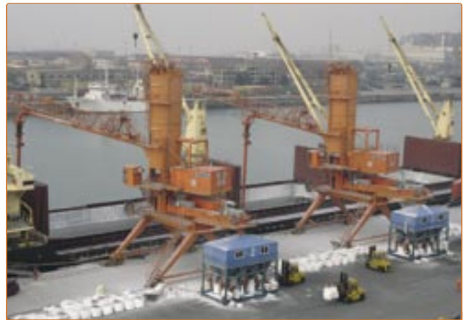
Figure 1. M300AL unloaders at Qingdao Port.
