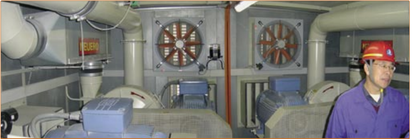
Figure 4. The Machinery House.
